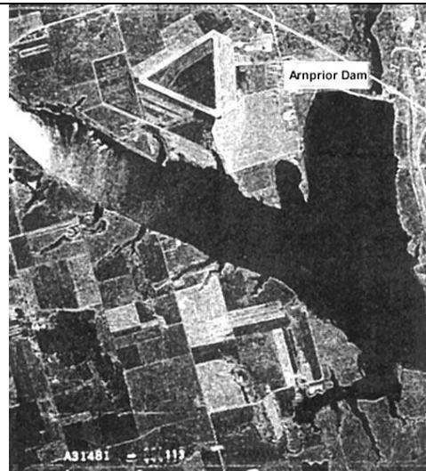
Figure 5 Arnprior Dam and Reservoir
