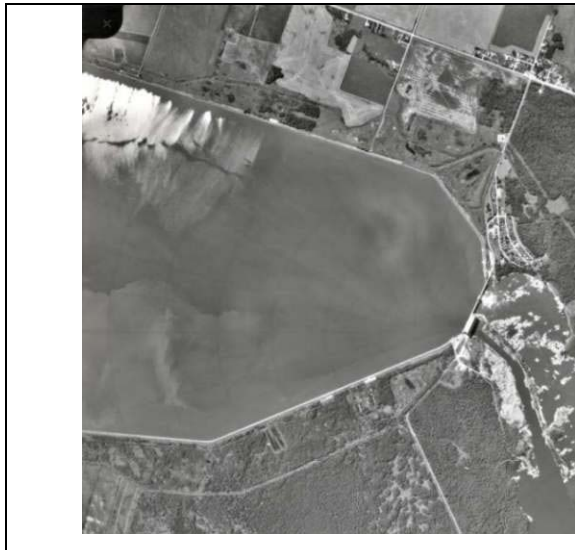
Figure 4 Seven Sisters Dam and Reservoir
