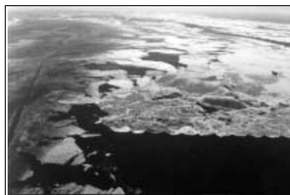
Figure 9: Triangular-Shaped Ice Accumulation “Dead Wedge” Upstream of the Yamachiche Boom Placed in Lac St. Pierre (in the St. Lawrence River)
