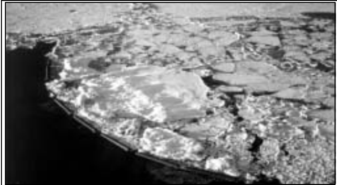
Figure 3: Lavaltrie ice boom. This is a close-up view of one 120 m wide span of the 1 km long Lavaltrie Ice Boom. The current velocity at this location is 0.8 m/sec
