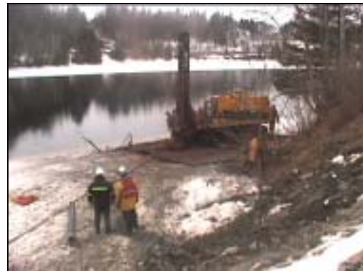
Figure 10: The drilling rig on the shore ice.
