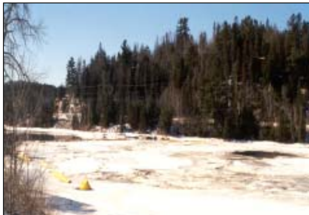
Figure 2: The accumulation of ice floes upstream of the ice boom 24 hours before the opening of the boom. This photo was taken on March 13, 2000.
