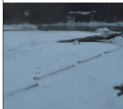
Figure 7: The snow behind the boom drifted 300 m to form a barrier and blocked the ice drift. Photos on December 12 and 20, 2000.
